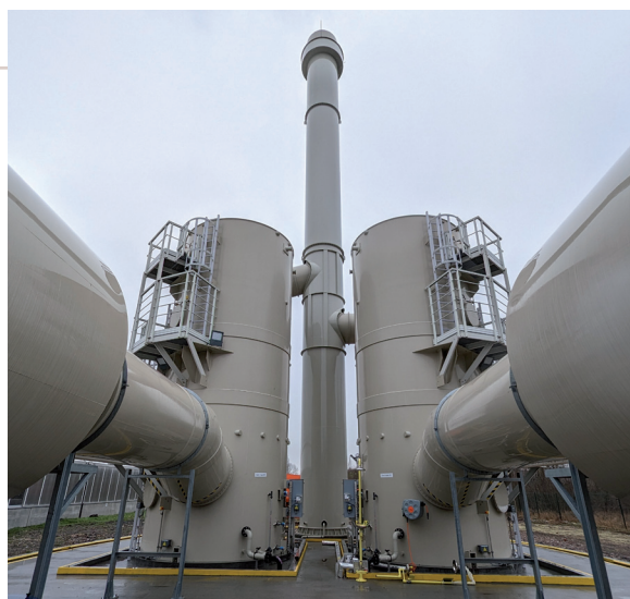
AyraScrub™ is an effective process for removing acid gases, VOCs and other pollutants from off-gases.
